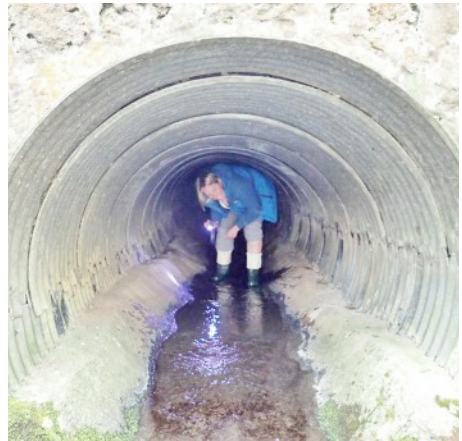
Exploring a culvert in Midlothian © Katty Baird
