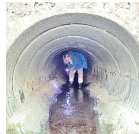
Exploring a culvert in Midlothian © Katty Baird
